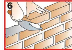
Spread mortar onto the header of the next, making a neat 10mm bed for the header joint. Press the brick against its neighbour, scooping off excess mortar with the trowel.
