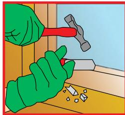
The process of cleaning out an old rebate to take new glass is known as hacking out. Wear protective gloves and goggles to remove segments of glass from the broken window. Use a hacking knife to hack out old putty and glass. Carefully pull out panel pins with pliers or pincers. Clean out rebate using a dusting brush.
